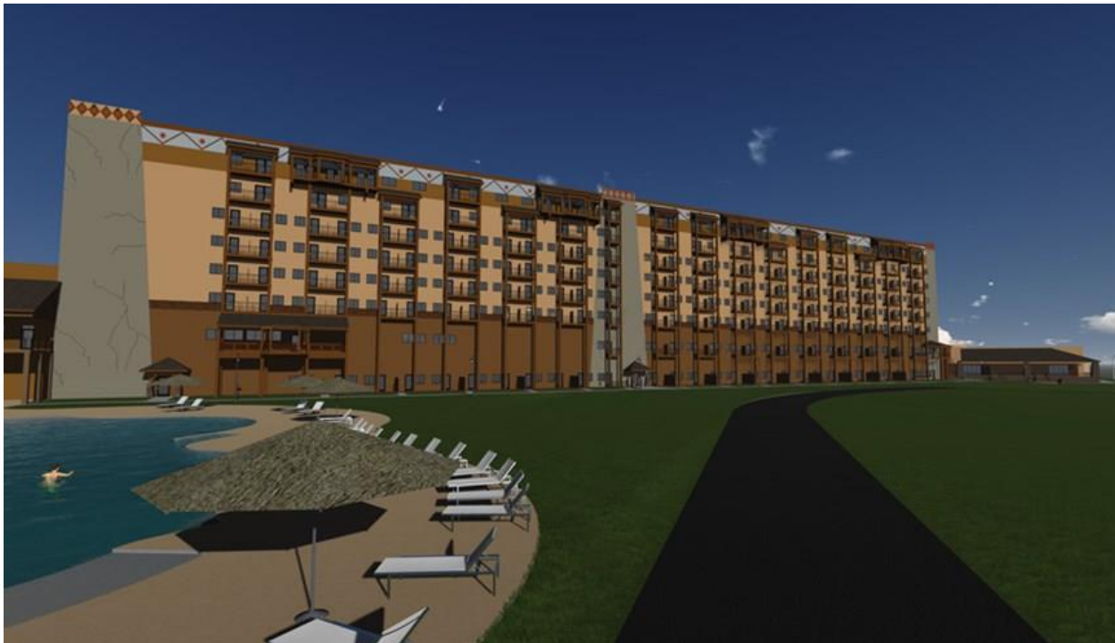
Figure 32 View of Hotel Building from South
